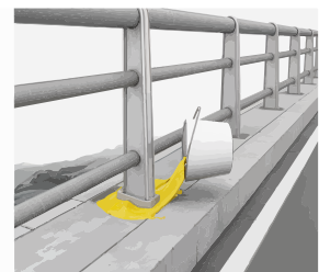
FILLING JOINTS IN PRECAST CONCRETE
